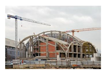
Scaffold was required on both theatre halls to undertake ceiling works, and plastering and coating works on lateral façades.
