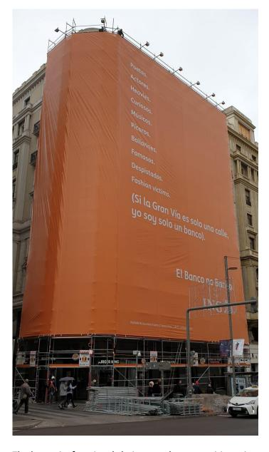
The key to its functional choice was the competitive price and the necessity to mount a 1.50 m wide passage frame to allow pedestrian crossing.
