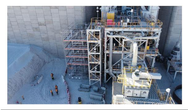
Problem: Catari's client, Cerro Nevado S.A., had to assemble an emergency stair tower box for Chancador Primario. To do this, they needed to generate scaffolding work areas around the entire perimeter to be able to assemble and weld the sections of the stair tower, which would be mounted as it rose in height. As there were no nearby structures for anchoring, a completely self-supporting scaffolding had to be built, reinforcing the high safety standards required by the mining company.
