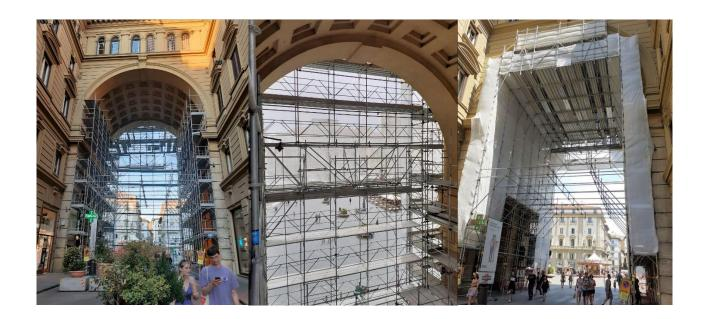
"Furthermore, the geometry of the structure was 'forced', the beam was designed using 250 and 180 cm modules, while the overhangs boulders were made with modules of 83 cm. This was made possible by the slight bending of the top truss which, although shorter than 1 cm per module (83 + 83 + 83 = 249) instead of 250, was easily 'closed' by the operators." Eng, Calvelli.
